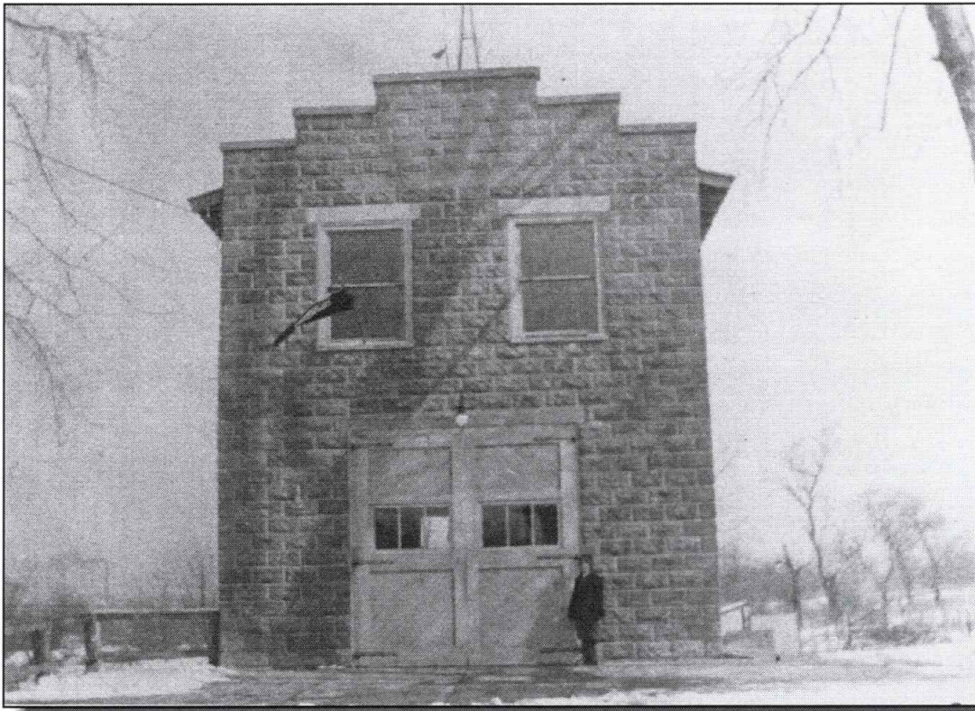
The completed firehouse as it appeared in late 1917 and early 1918. Note the swing-open doors.
