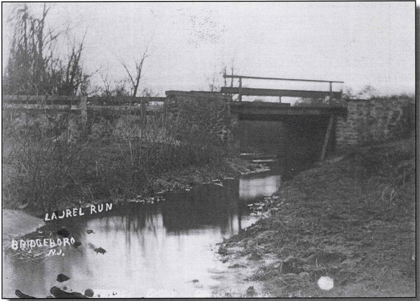
Laurel Run was dammed where it ran under Bridgeboro-Moorestown Road and here at Creek Road by our firemen. Prior to the installation of fire hydrants in the late 1960s, these ponds were created and needed to establish a drafting point for water supply.
