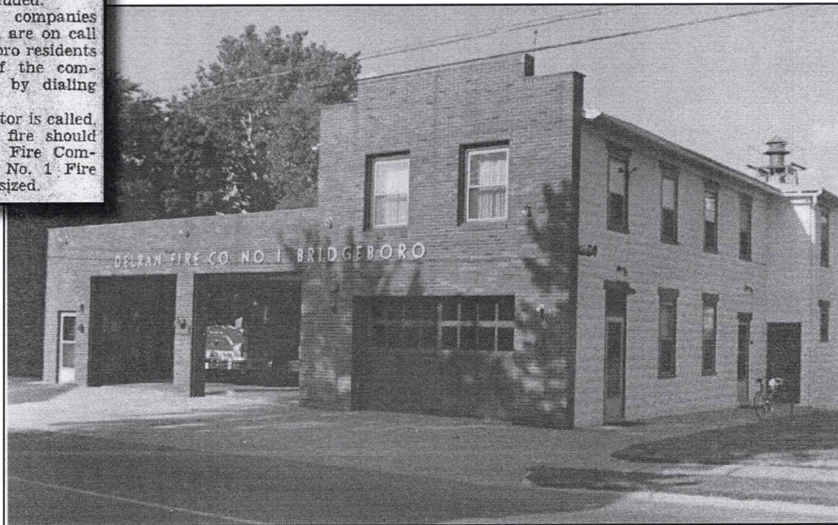
Our new addition completed. Note: In 1925, the two story addition was added to the rear of the original firehouse. (From the door on the side to the rear)
